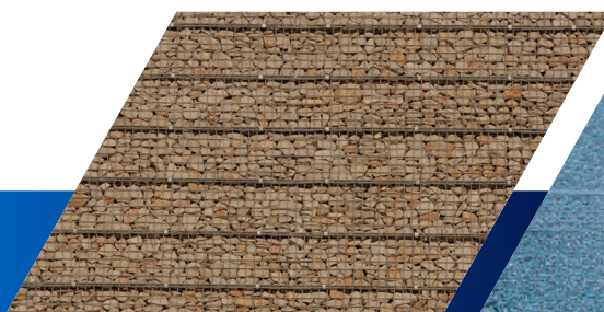
Vertical wire mesh facing
