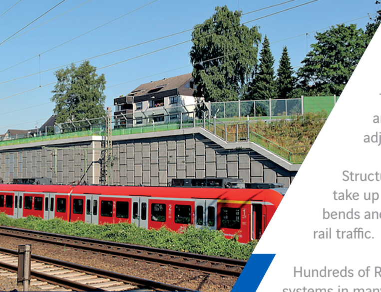
Haan-Gruten noise absorbing wall - Germany
