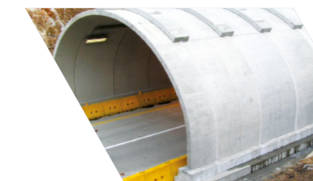
Tunnel extension - Hyeongok (South Korea)
