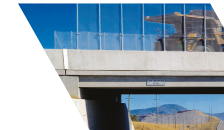
Bridge Abutment - New South Wales (Australia)
