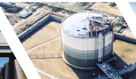
Containment dikes for ammonia tanks - Montoir (France)
