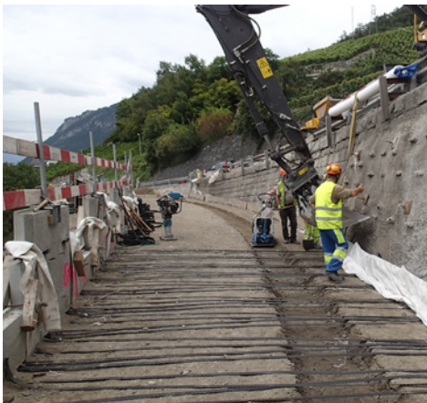
Friction Link system with synthetic strips
