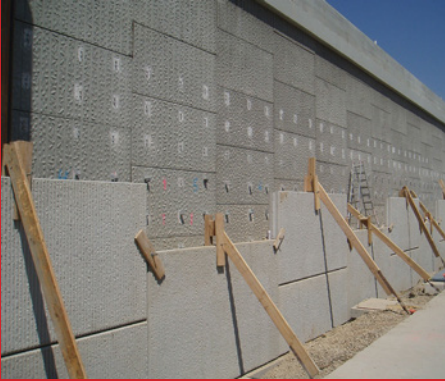
I-215 On-Ramp to Southbound I-15 Ramp widening, Salt Lake County, Utah, USA
