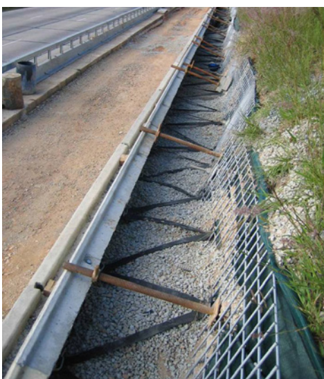
Direct Link system with synthetic strips
