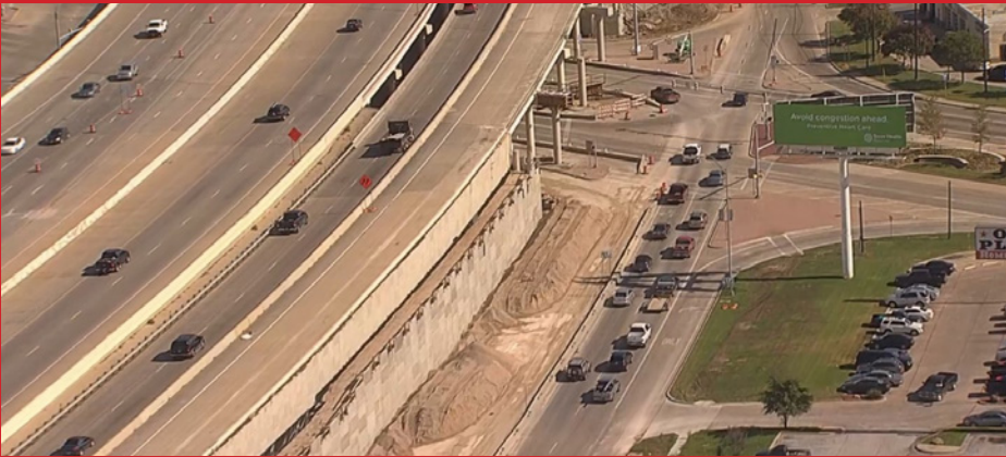
North Tarrant Express near Dallas, Texas, USA
