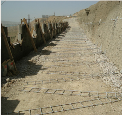
Friction Link system with steel strips
