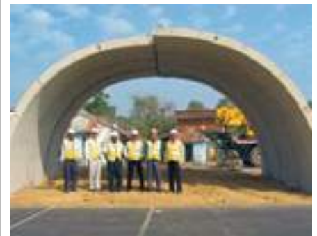
The RECo-India project team posing in front of segments of a partially built arch for an animal underpass.
