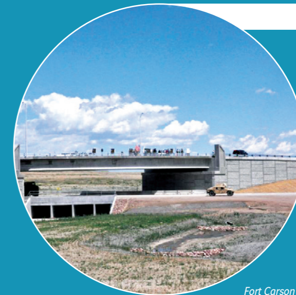
Fort Carson access road - Colorado, USA
