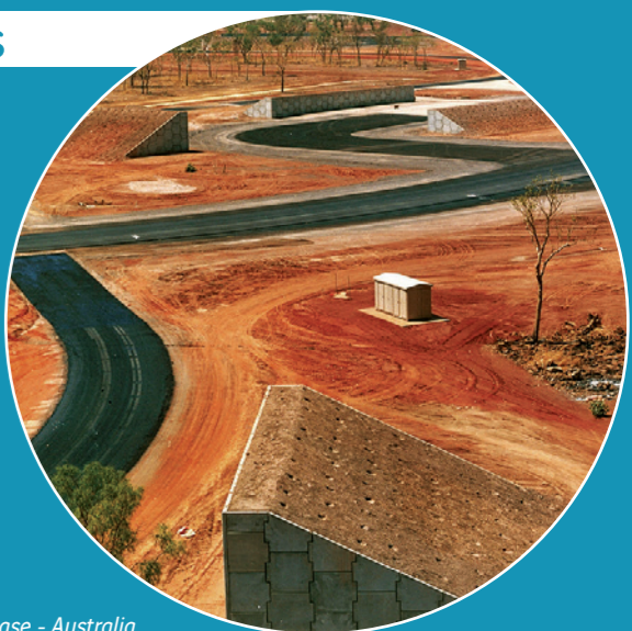
Blast protection air base - Australia
