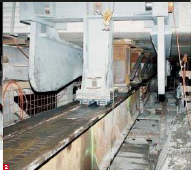
After being transported from the prefabrication site by a 180 t-capacity gantry crane, the new cover slab is placed on the sliding equipment installed at the south opening of the tunnel. The sliding operation, over 6 m, only takes place once the new slab is assembled and 'bonded' to the old one. Right: view of the runway moved after 4 launching operations.
