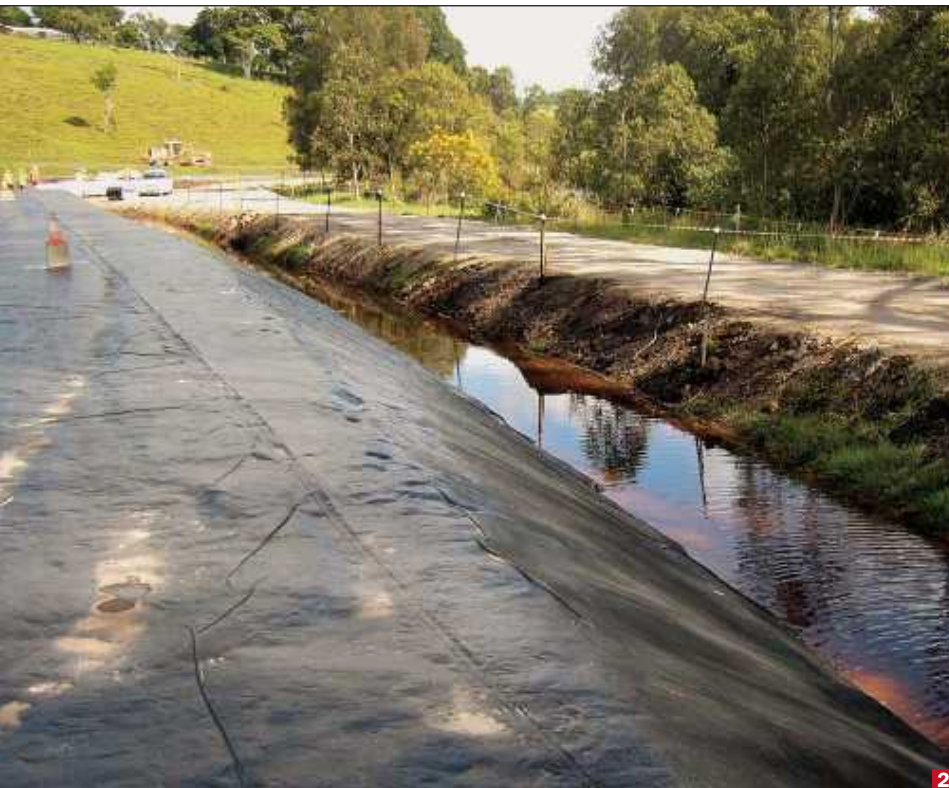
The Menard Vacuum process is an atmospheric consolidation technique used, like preloading, to consolidate saturated compressible soils with low permeability (clay, silt, peat etc.). It consists of installing a vertical and horizontal draining and vacuum pumping network in the soil to consolidate. The system is covered with an impermeable membrane (1) and surrounded by peripheral confinement trenches that anchor the impermeable membrane and ensure the soil to be consolidated remains saturated (2). The depression created by the pumping system (3 and 4) under the impermeable membrane means atmospheric pressure can be applied to the soil, with general values reaching – 60 to – 80 kPa depending on the overall system performance (equivalent to the preloading of 3 to 4 m of fill surcharge).
