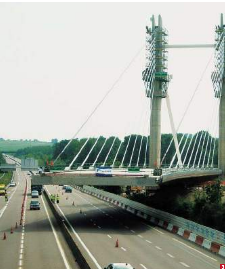
The 30 to 80 m long cables were adjusted using Freyssinet's Isotension system.
